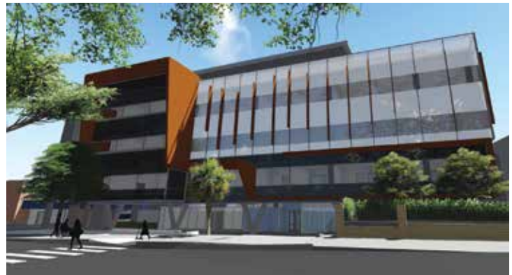
TOP: DR DAVID HAYES AND BRISBANE BULLETS PLAYER CAM BAIRSTOW ABOVE: ARTIST IMPRESSION OF BRISBANE PRIVATE HOSPITAL EXPANSION FRONT PAGE: DANNY DALTON IN THE NEW PAED WARD
